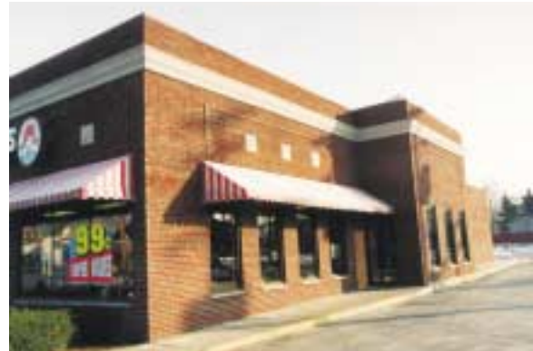
A pre-cast cornice installed just below the roofline adds architectural detail to the building's exterior.
