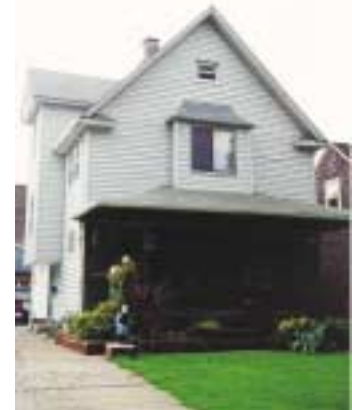
Alteration of second floor window configuration has disturbed the balance between wall space and window space on the front of the home.
