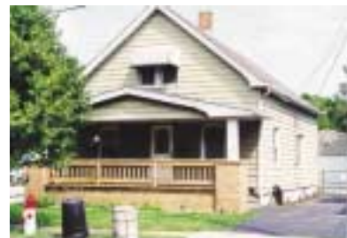
Non-original balustrade looks architecturally inconsistent with the house.
