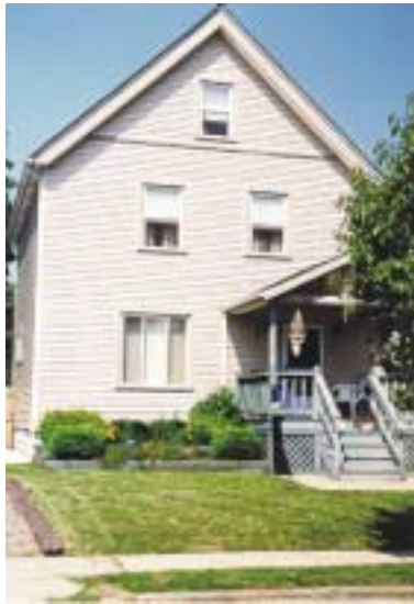
Sliding window installed on the first floor appears architecturally inconsistent with the other windows on the front facade, which are double-hung.
