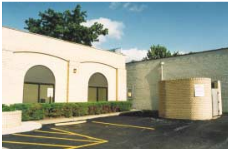
Although located in the front of the building, the exterior material of the walls of this trash storage area matches that of the main building. The enclosure is well constructed so that it completely hides the trash dumpster located inside.
