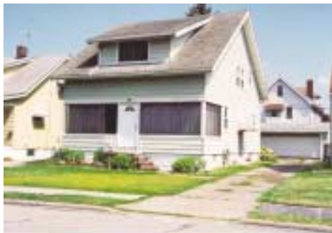
Roof shape: side-facing gable
