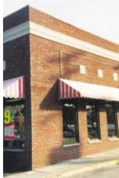
Examples of tile and pre-cast stone (concrete) set in brick
