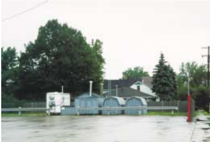
At left, mechanical equipment is completely exposed to public view
