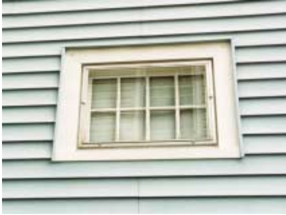
Exposed window frames
