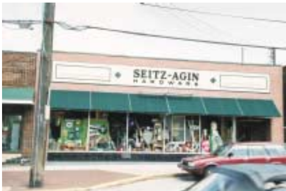
Signage in building's lintel area
