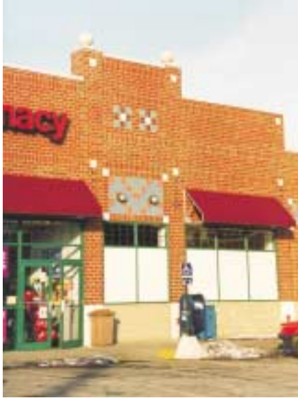
Examples of tile and pre-cast stone (concrete) set in brick
